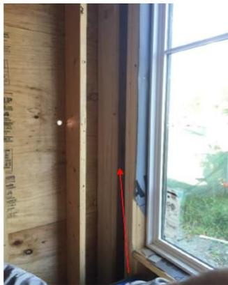
*The wall to the left of the corner will be spray foam and the wall to the right will be cellulose. Instead of putting cellulose in the first bay (red arrow), put spray foam there instead. It will connect the spray foam air barrier directly to the backside of the taped sheathing air barrier.*
