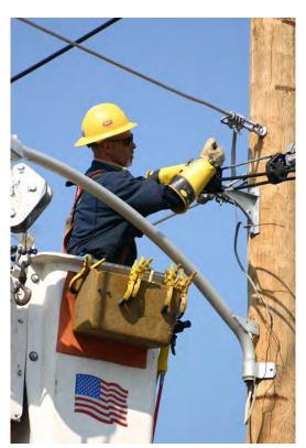
aerial circuits by converting 4.16 kV circuits to 13.8 kV, and upgraded switches, reclosers, and communications equipment to allow remote switching.
