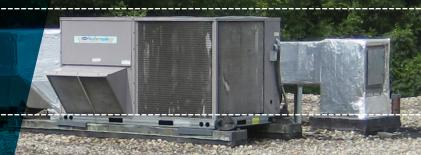
Rooftop units heat, cool, and ventilate commercial facilities such as office and retail spaces, grocery stores, and restaurants. Standard rooftop unit fans operate at full speed at all times. This wastes a considerable amount of power when your building isn't experiencing extreme temperature highs and lows—which is more than 90% of the time.
